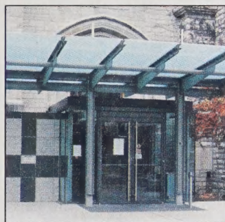
The entrance to the new Douglas Library
